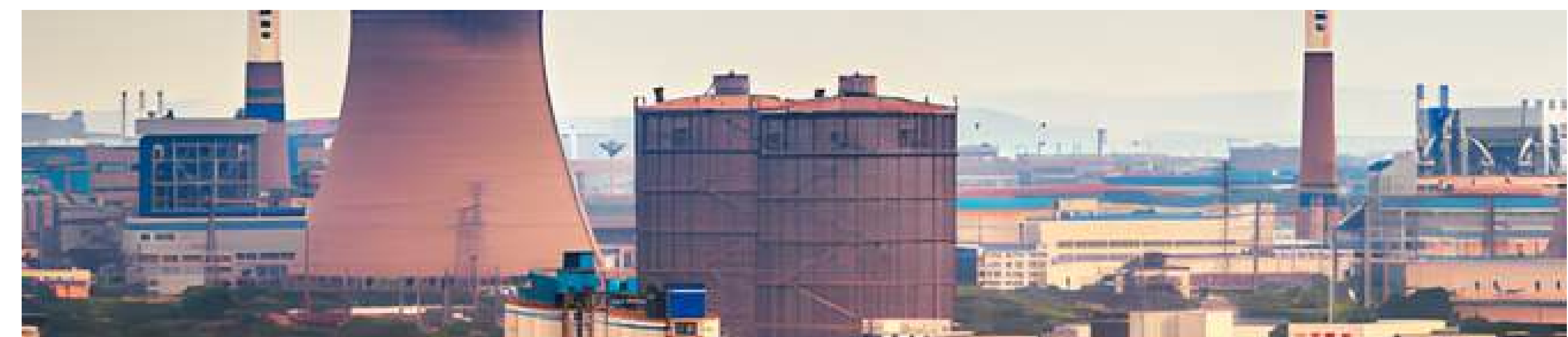
► Corrosion Failure Analysis of Industrial Equipment
